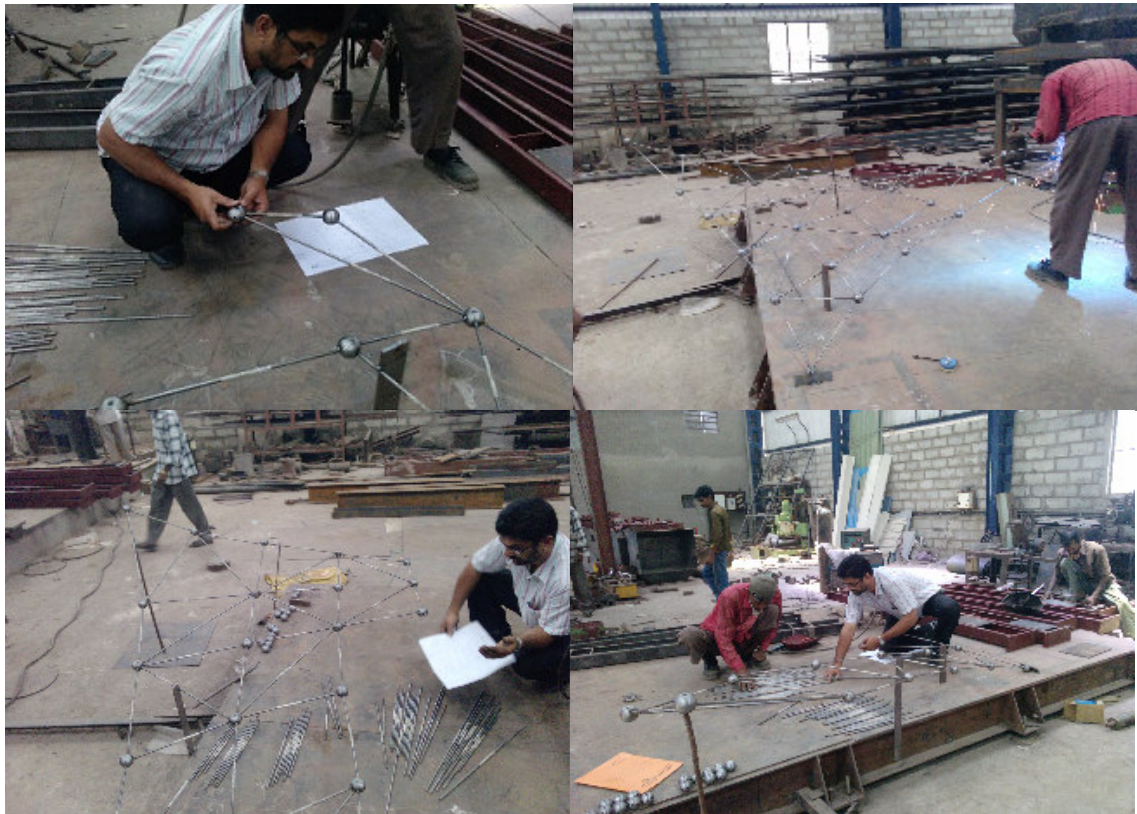
Figure 4: Small steel roof prototype fabrication & assembly
