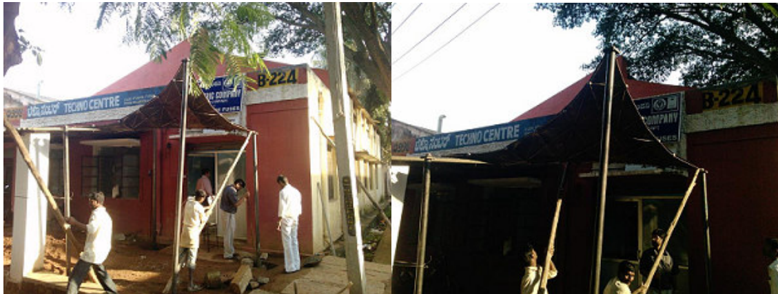
Figure5: Small steel roof prototype installation
